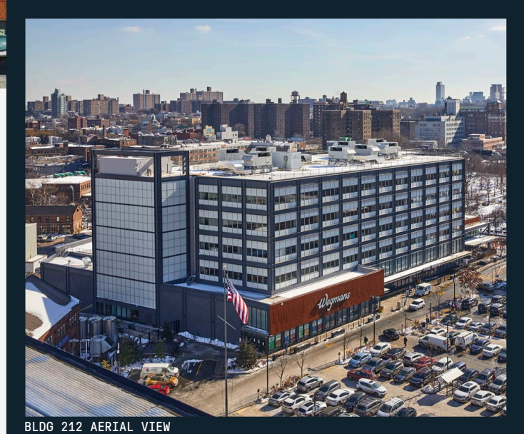
BLDG 212 AERIAL VIEW
