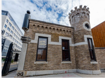
SANDS ST. GATE / KINGS COUNTY DISTILLERY
