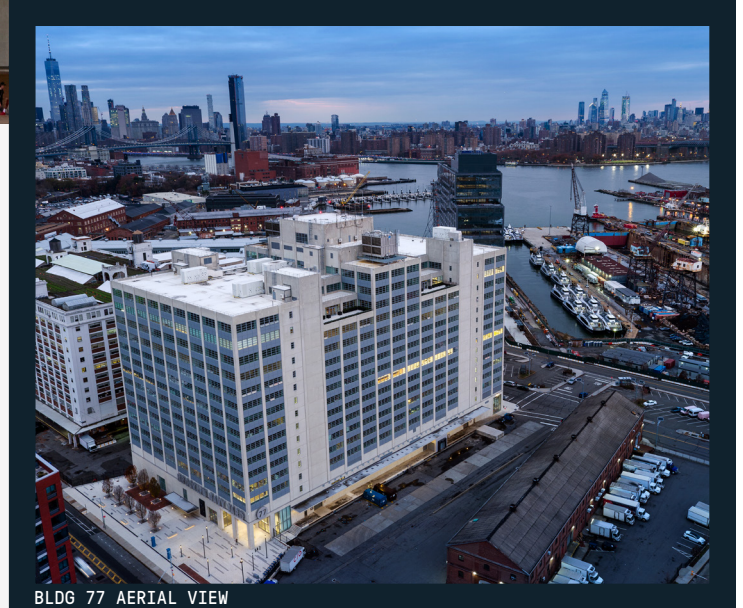
BLDG 77 AERIAL VIEW
