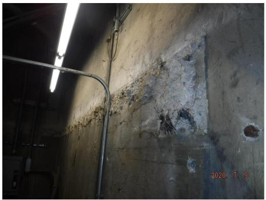
Electrical Room: Non-asbestos containing miscellaneous tar on wall.
