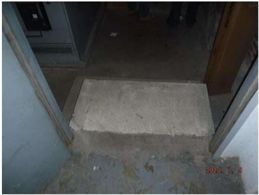
Electrical Room: Lead containing blue paint over concrete floor in vestibule.
