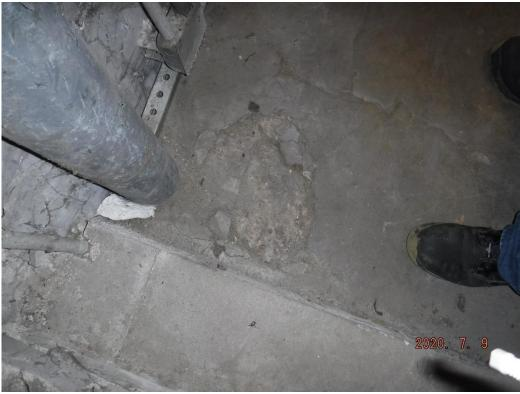
Electrical Room: Non-asbestos containing lightweight concrete floor.
